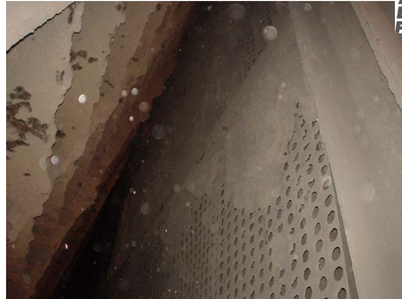
Lower Precipitator Inlet Flow Distribution Plates Gavin 1 - 5/17/04
